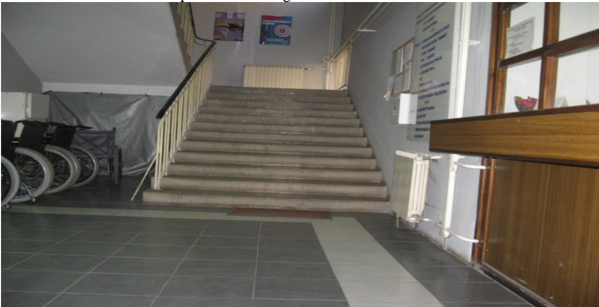
Stairs that lead to other floors in the building
