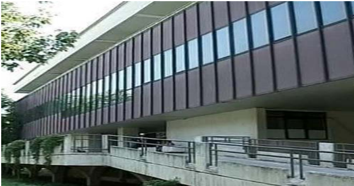
The building of Clinic for Plastic and Reconstructive Surgery- Skopje
