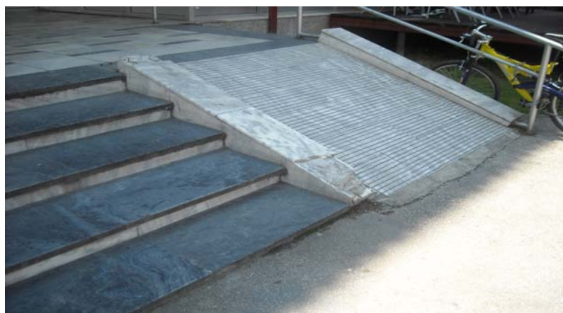
Figure 2.1. The ramp at one of the entrances
